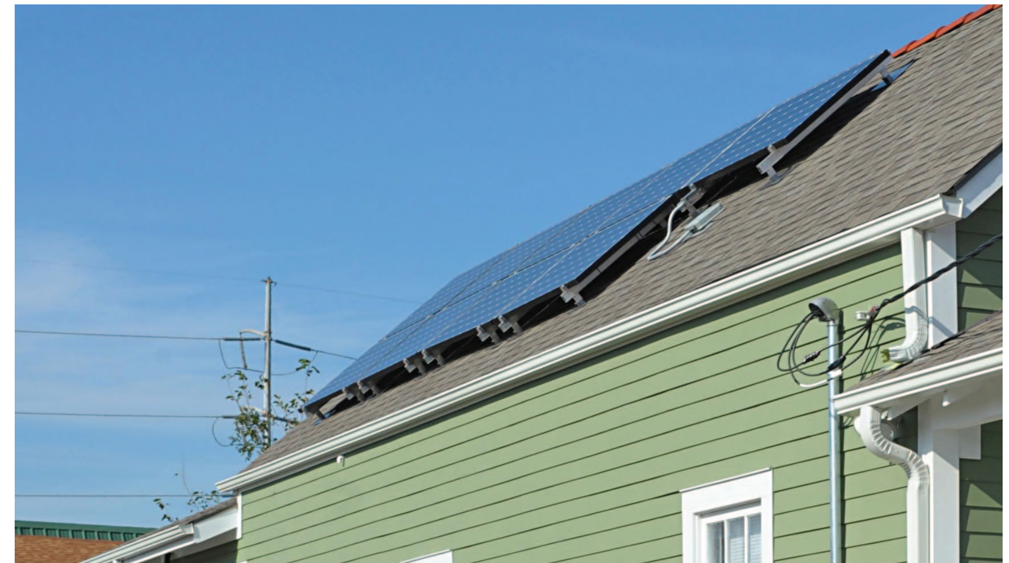
SOLAR PANEL @ 8522-8524 PLUM ST
