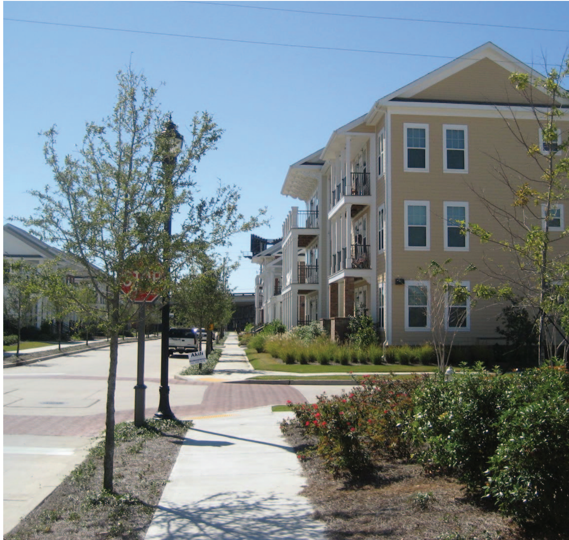
COLUMBIA PARC, NOLA (SAINT BERNARD REDEVELOPMENT HOUSING PROJECT)
