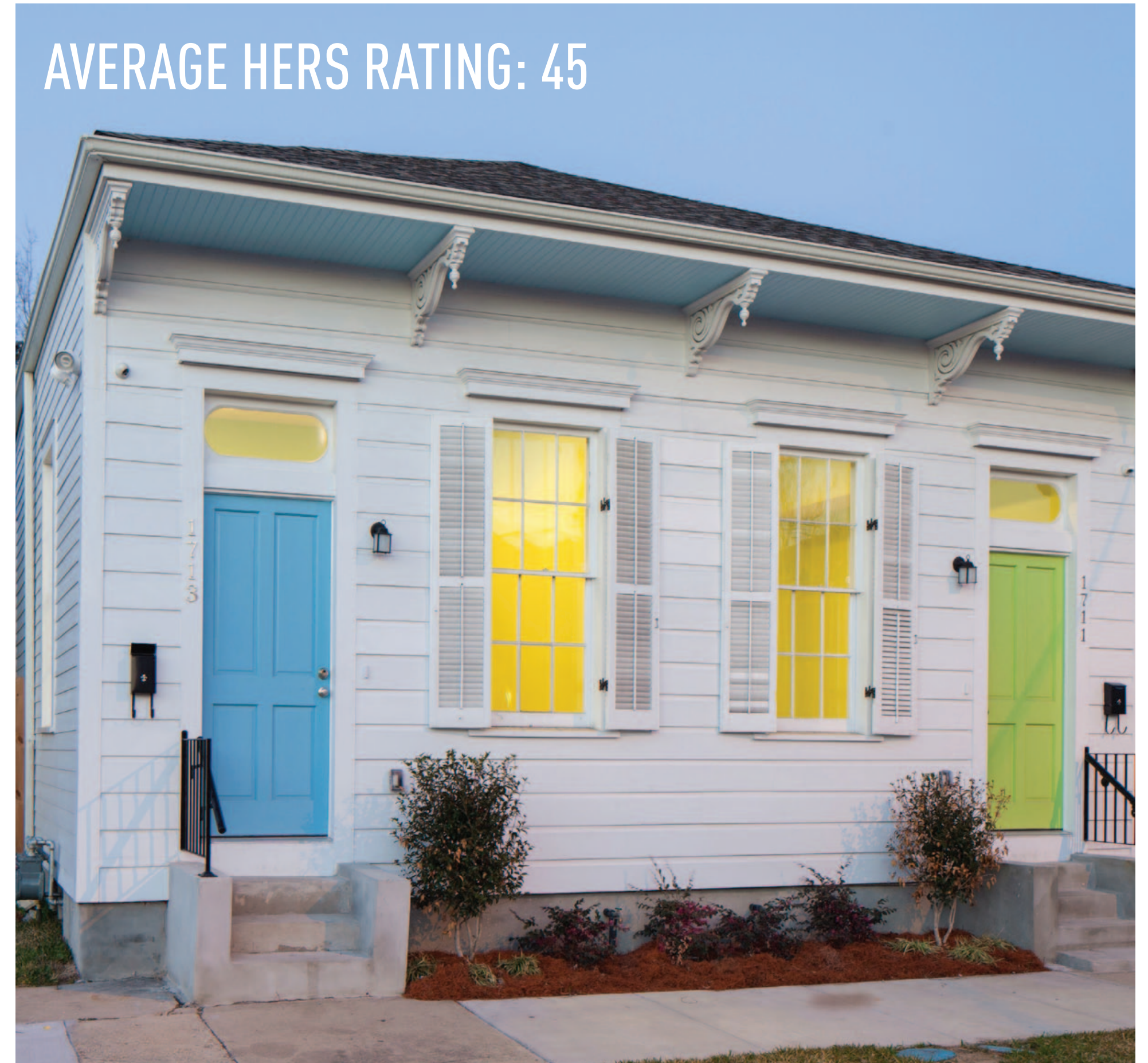
BLOWN CELLULOSE INSULATED RESIDENCE
